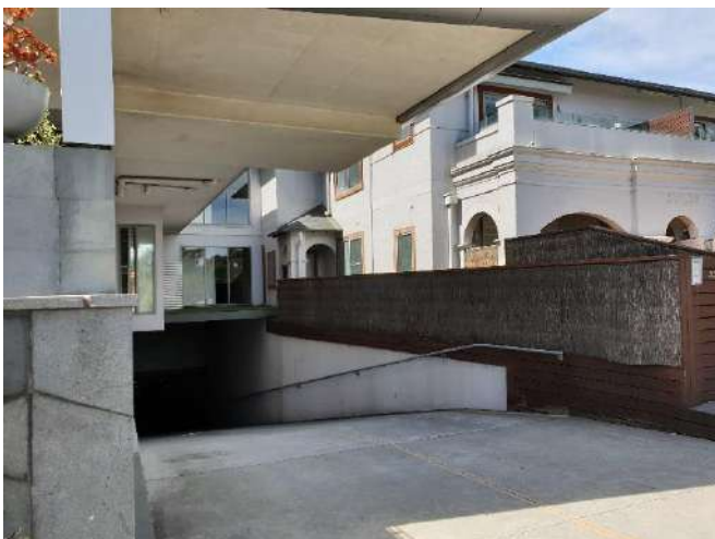
Basement Entry Ramp
