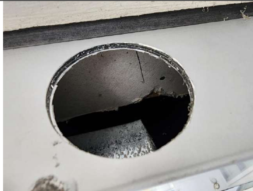
Sample 1, ACP, Unit 24, level 1, south elevation
