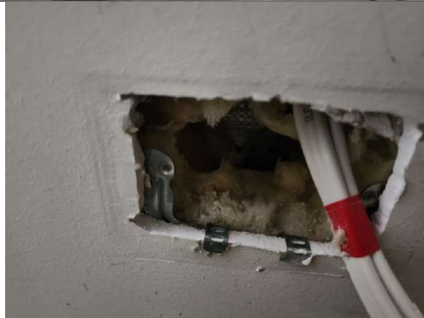
Sample 2, insulation, concrete wall, Unit 24, west elevation
