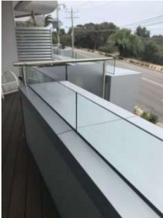
Typical configuration of ACP provided to the leading edge, capping and small downturn on the inside face of the balustrade.
