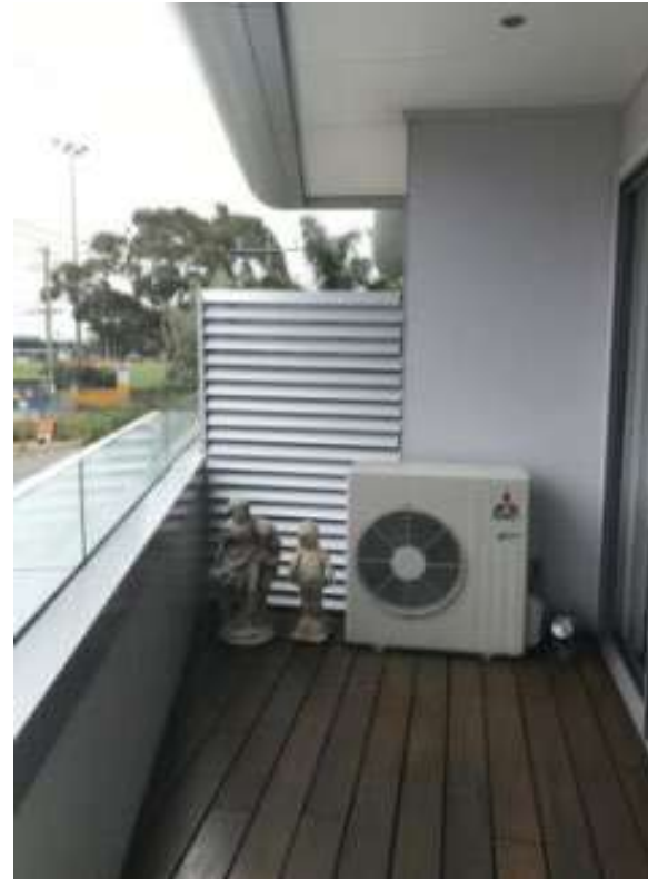
Typical configuration of ACP provided to the leading edge, capping and small downturn on the inside face of the balustrade.
